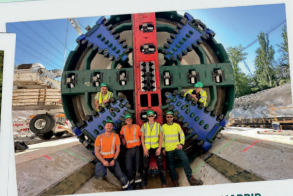
OVERSTROMINGSWATER TUNNEL, MADRID
