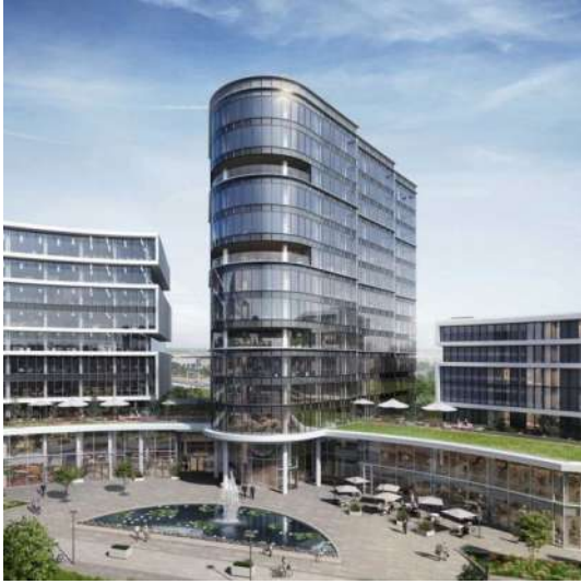
Airport Business Center Diegem
