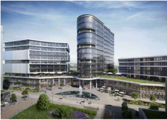
Airport Business Center Diegem
